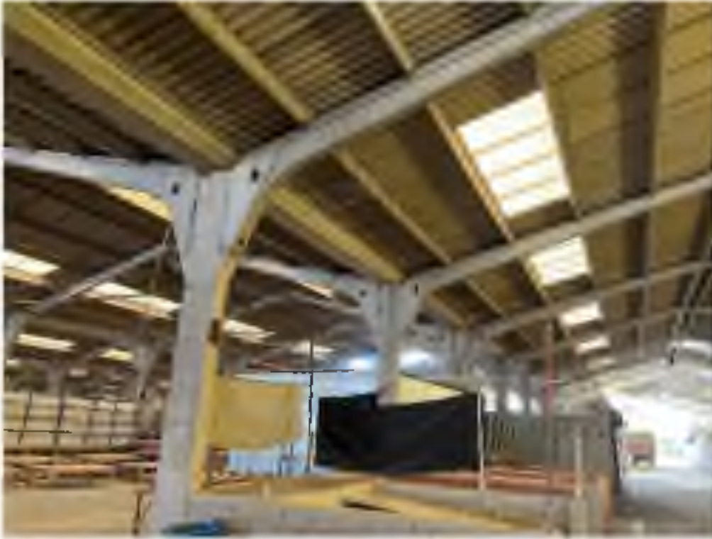
An Inside View of Rooftop
