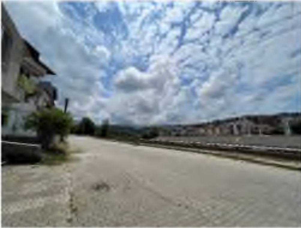
Keskin Street at East
